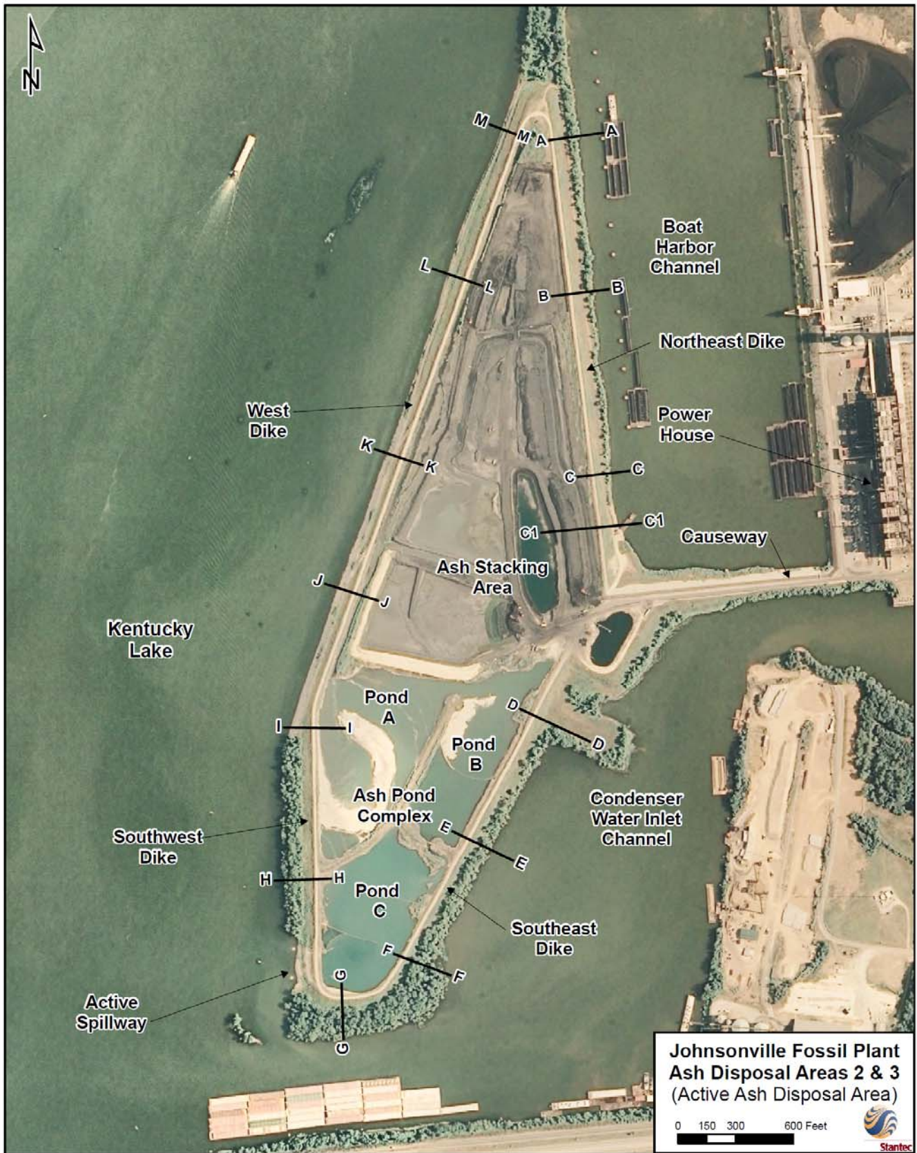
Figure 1. Ash Disposal Areas 2 and 3
